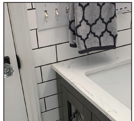
Door jam (no additional edge required)
